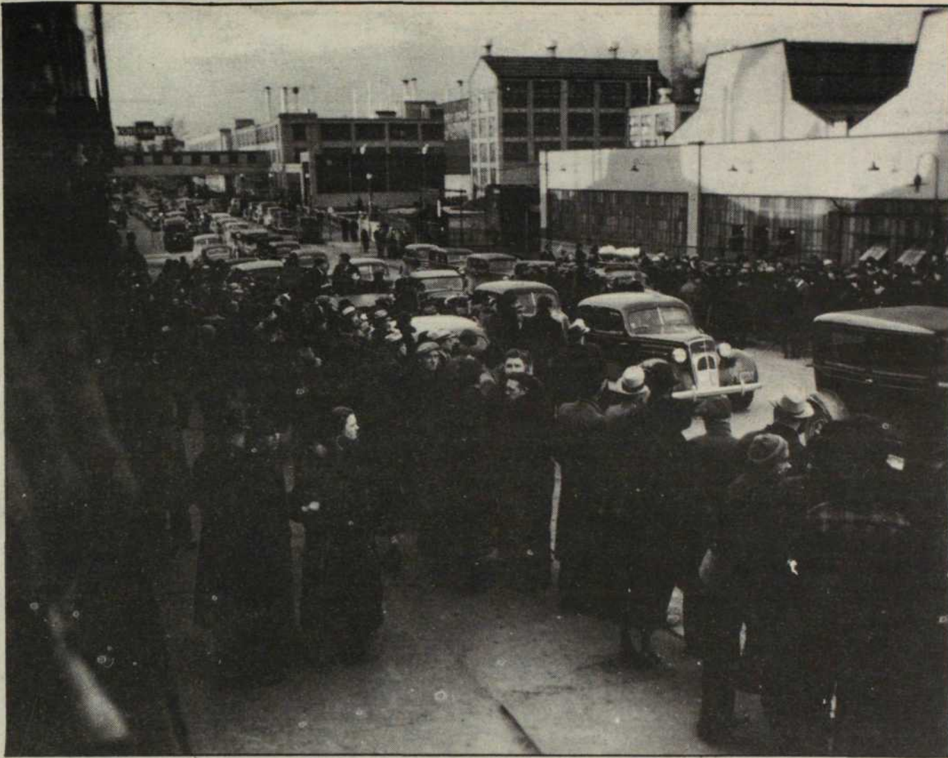
Shortly after this picture was taken of Plant #4 on Feb. 1, 1937, the diversionary attack at Plant #9 allowed strikers to seize Plant # 4 and thus to effectively shut down all of General Motors Chevrolet Production.
